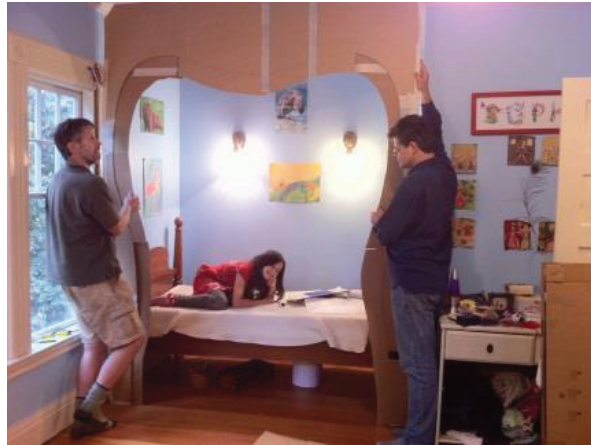
Figure 6: Step 1 - Mocking up the alcove opening.
