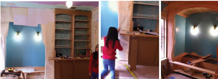
Figure 12: Step 6 - Mocking up the vertical shape “legs” of the alcove opening.
