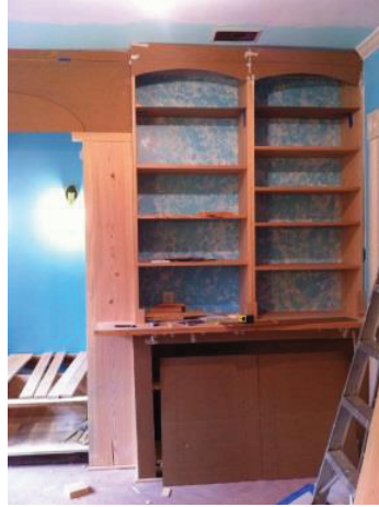
Figure 11: Creating a vertical spine with inner alcove shelving.
