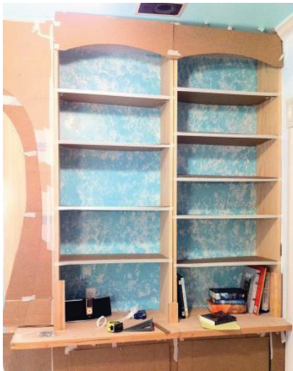
Figure 13: Mock-up Shelving and Top Arch Shape and shelves.
